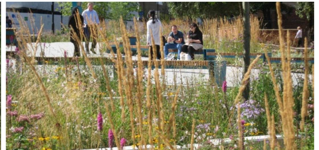
The sustainable urban drainage system frames public seating areas
