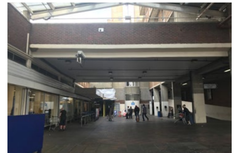
The shopping centre lacks diversity and a contemporary offer.
