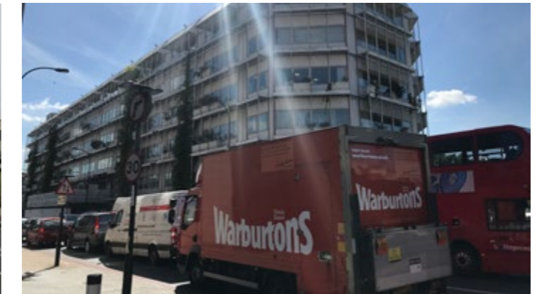
12. Catford Road is congested and severs the town centre
