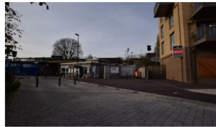
07. The Catford station building is underwhelming
