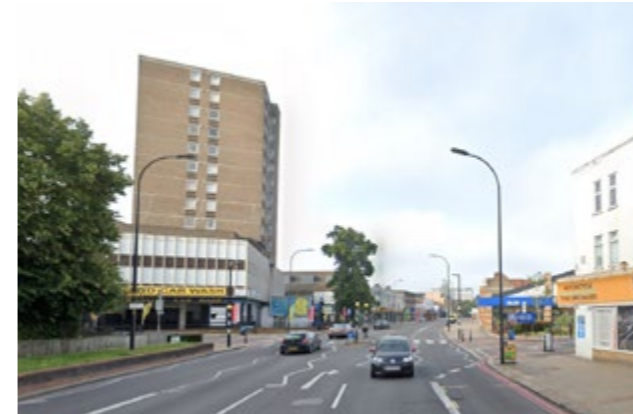
The single storey to the right does not feel like a town centre
