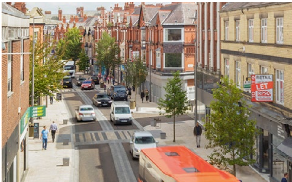
A town centre high street with pedestrian priority and traffic calming.
