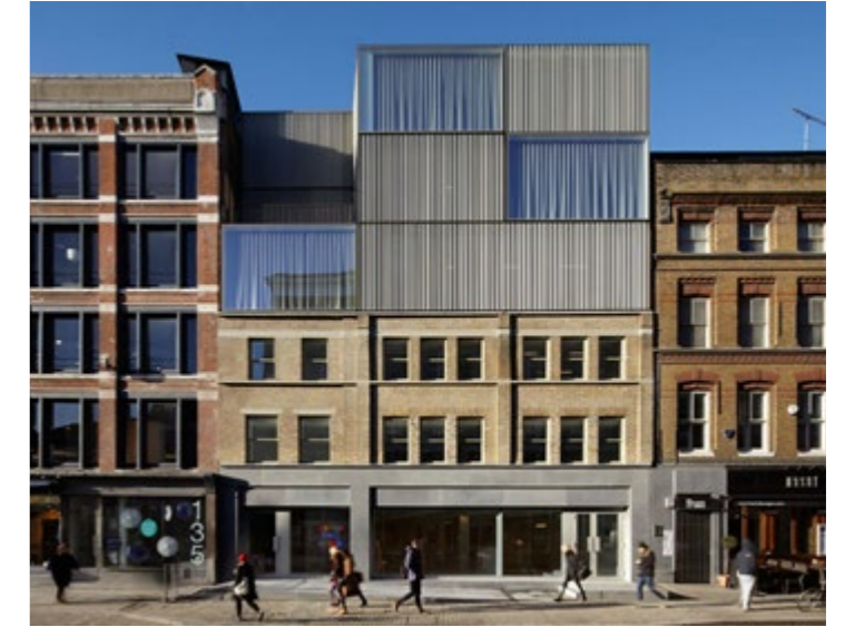
Existing traditional materials are complemented by contemporary architecture
