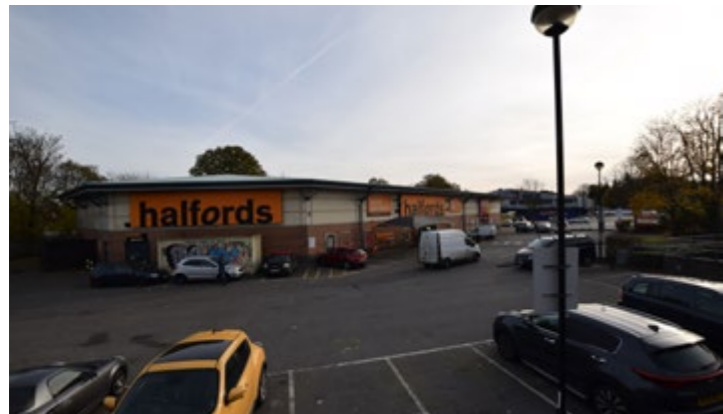
03. The Wickes & Halfords site is underutilised and cut off from the town centre
