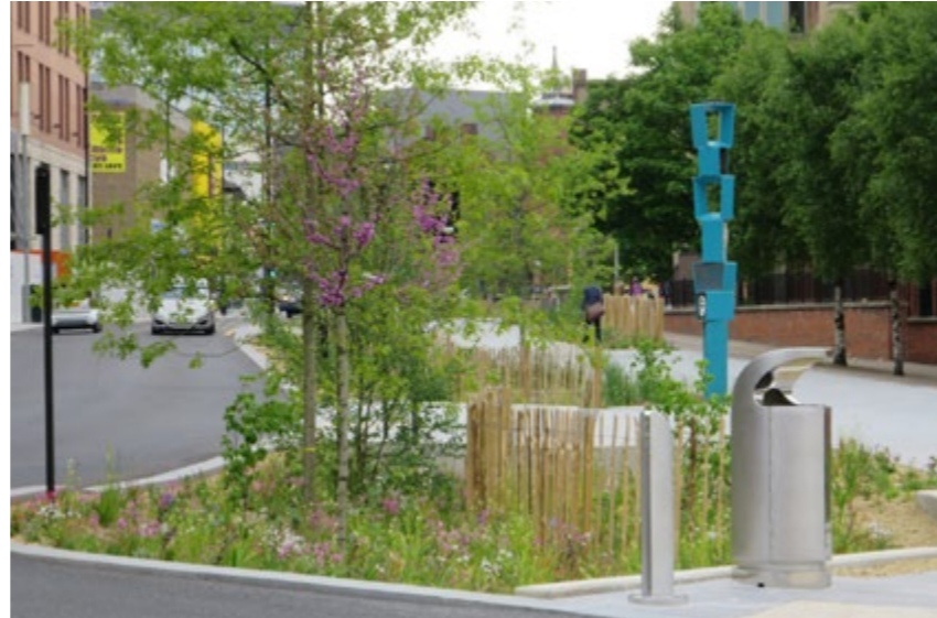
Public art is integrated into the sustainable urban drainage system
