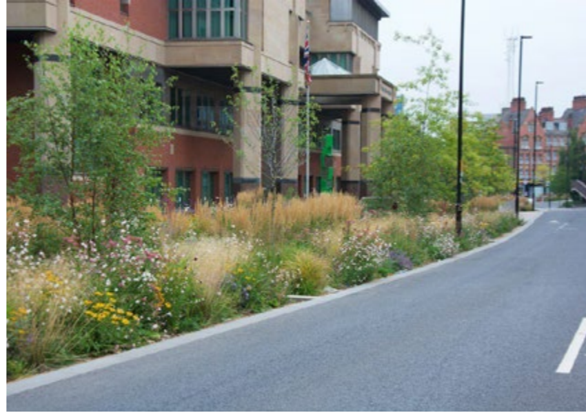
Swale plant bed as part of sustainable urban drainage system in Sheffield
