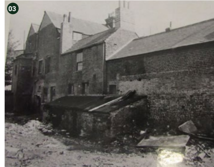
Elmwood Farmhouse (Catford Constitutional Club) - locally listed
