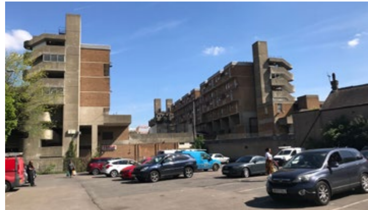
02. Surface car parking cover several underutilised town centre sites
